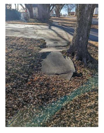
Sycamore Street (looking south towards 3<sup>rd</sup> Street) - Broken sidewalk caused by a tree
